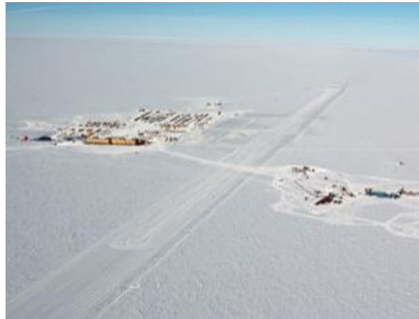
Picking up the pieces - the IceCube facility at the South Pole (Image: Forest Banks/NSF)
